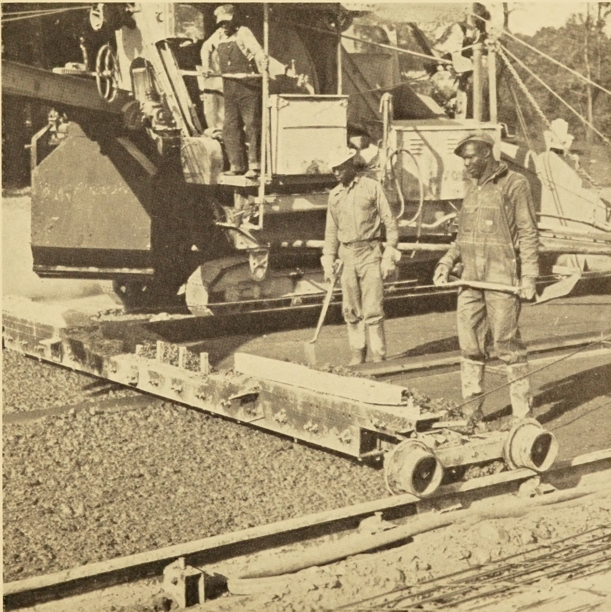
CONSTRUCTING EXPERIMENTAL CONCRETE PAVEMENT IN INDIANA
